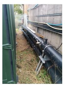
Figure9: mine water being tapped for the pilot plant from the main line
