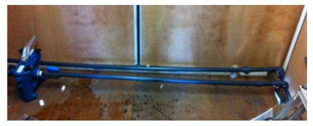
Figure 14: A duplex filter to remove ochre and other suspended particles
