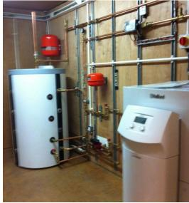
Figure 6: Heat pump and the Buffer tank
