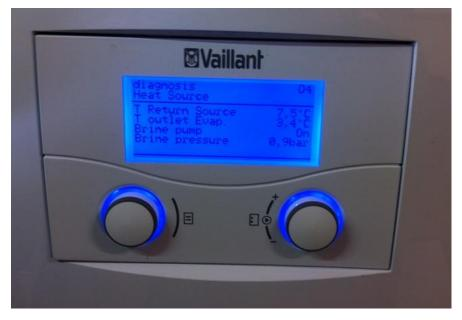
Figure 11: Heat pump diplaying the brines temperatures
